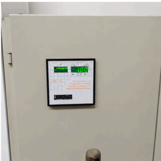
Power Factor Correction Unit – Mains
