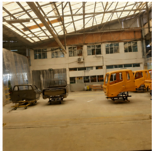
Daylighting via Clear Polycarbonate Sheets
